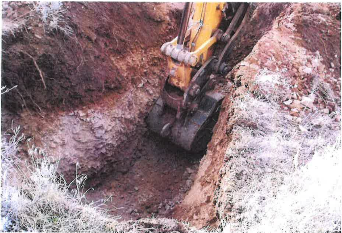
Test Pit TP-03
