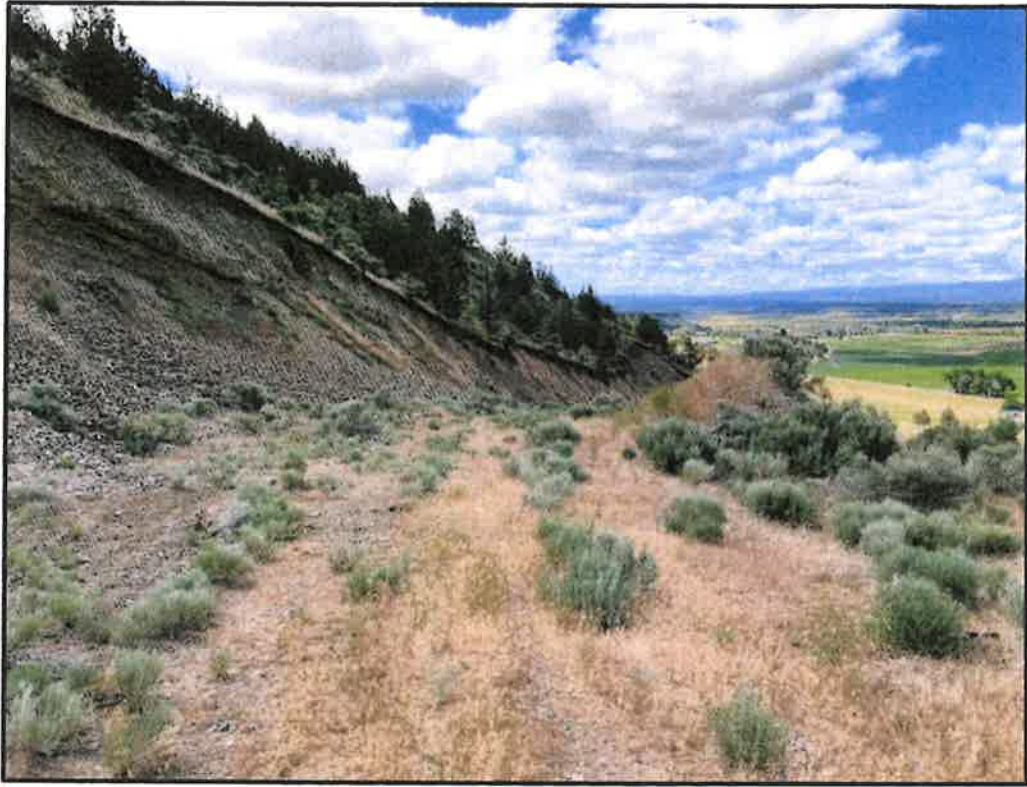
View looking southwest at existing road cut.
