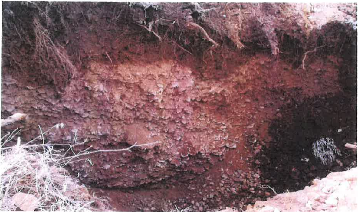
Test Pit TP-03
