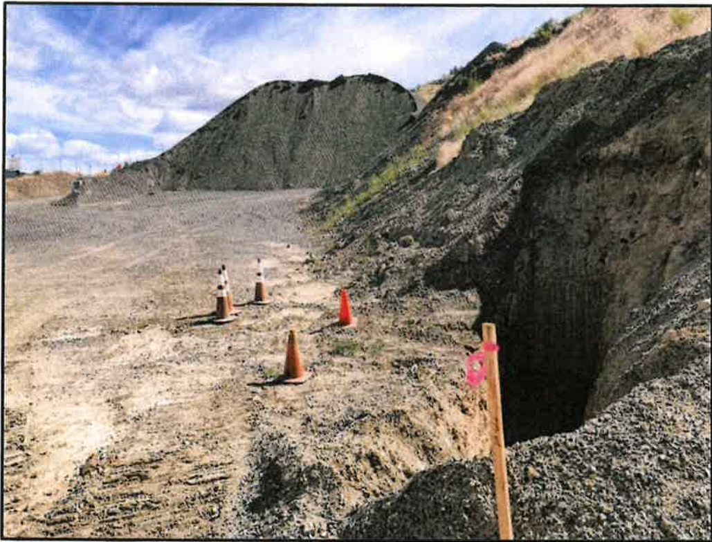
TP-01 at photo right. Note overburden silty sand overlying talus/screed unit. \frac{3}{4} " stockpile in background.
