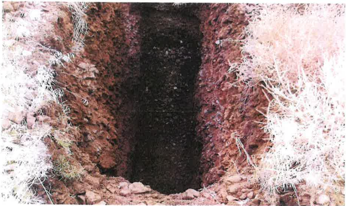
Test Pit TP-06
