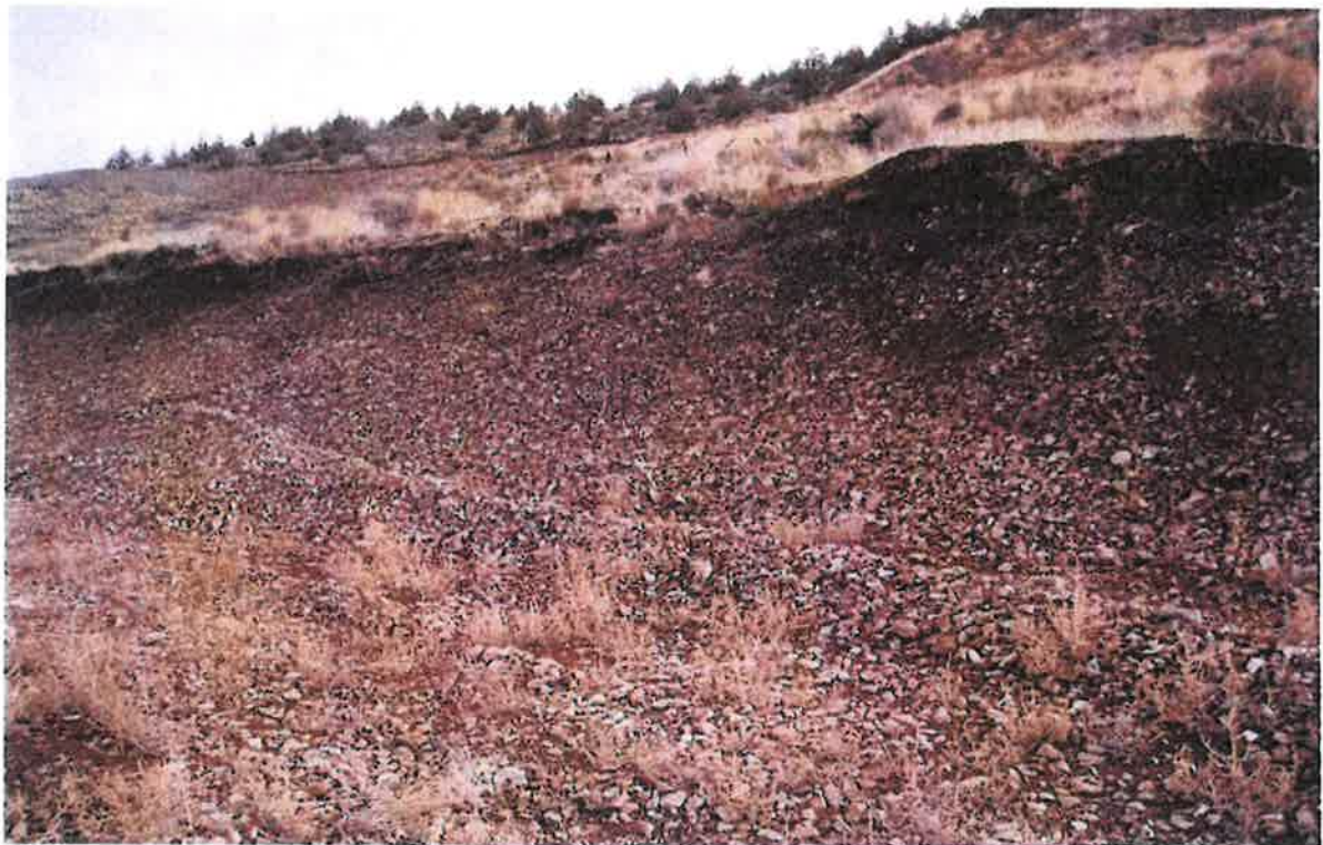
Upper terrace cut face
