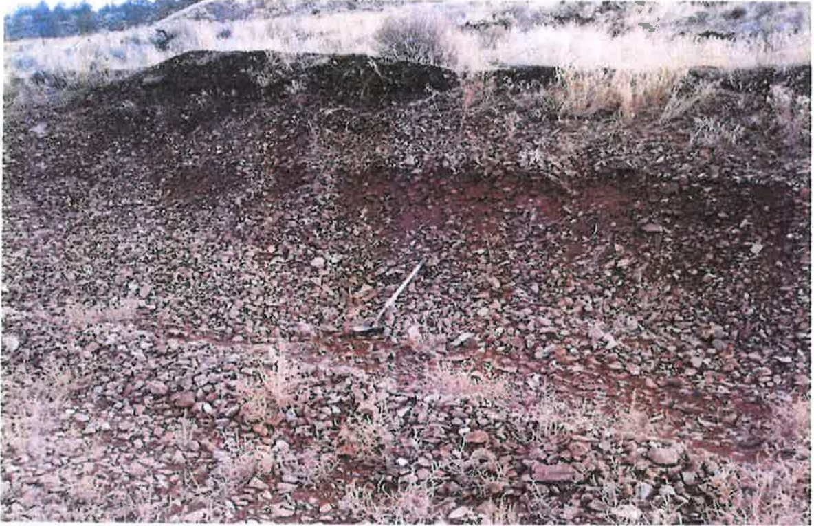
Upper terrace cut face above TP-05
