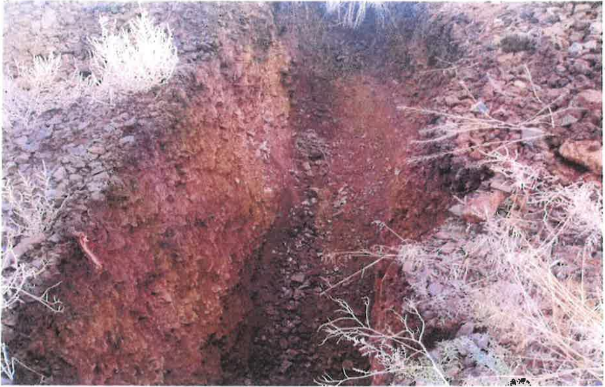
Test Pit TP-01
