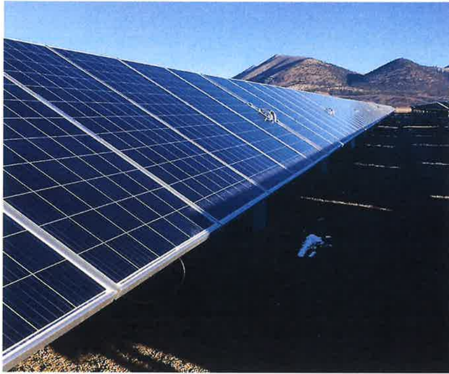
Figure A-3 – PV Module Array strings on single axis tracking racking (central OR)
