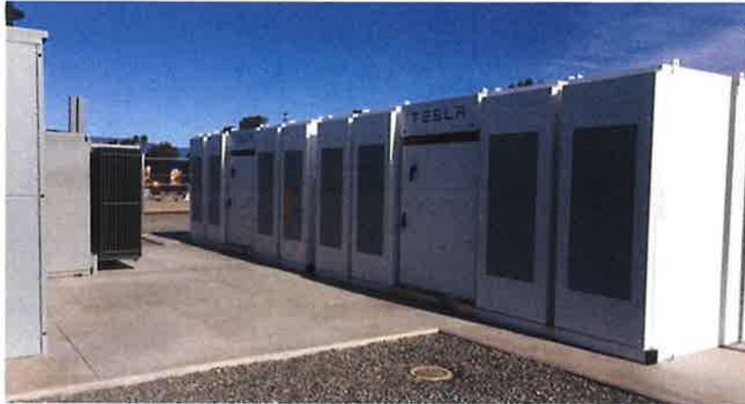
Figure A-5. Example inside substation, showing modular energy storage equipment, 34.5 kV transformers, breaker cabinets, and ancillary equipment on concrete mounted pads.
